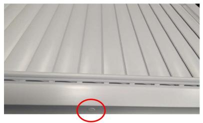
**Note:** The placement of the caps may be either above or below the centre point, depending on the number of louvres and positioning of handle rebates and mid-rails.
